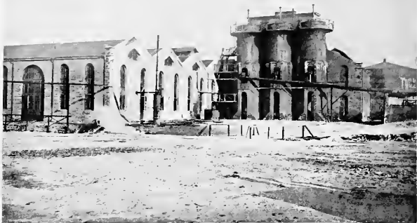
PARTS OF THE REFINERY OF THE SCHIBAIIEFF PETROLEUM COMPANY (LONDON), OF WHICH MR. J. CATER SCOTT IS CHAIRMAN. MOST THOROUGHLY UP-TO-DATE AND THE LARGEST BRITISH-OWNED REFINERY AT WHITE TOWN. THE TOP VIEW SHOWS THE CONTINUOUS LUBRICATING OIL PLANT, WHICH CONSISTS OF 12 STILLs, EACH OF 20 TONS CAPACITY AND TAKING A CHARGE OF 10½ TONS. THIS DEPARTMENT OF THE REFINERY DISTILLS FROM 355 TO 420 TONS OF MAZOOT PER DAY, AND PRODUCES 100 TONS OF SOLAR OIL, 16 TONS OF SPINDLE OIL, 90 TO 105 TONS OF ENGINE OIL AND ABOUT 10 TONS OF CYLINDER OIL. THE SECOND PHOTO SHOWS THE REFINING DEPARTMENT OF THE LUBRICATING OIL PLANT, WHICH IS CAPABLE OF PRODUCING UP TO 160 TONS OF ENGINE OIL PER DAY.
