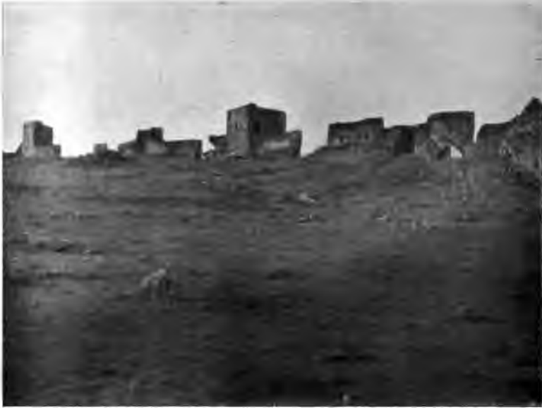
ANI. WALLS VIEWED FROM WITHIN.
