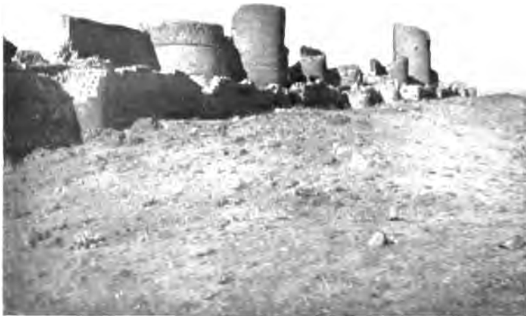
ANI. THE WALLS VIEWED FROM OUTSIDE.
